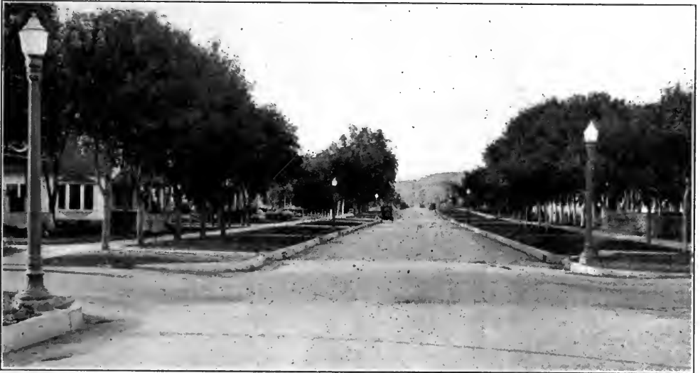
LIGHTING UNITS ON RESIDENTIAL STREET, MANDAN, N. DAK.
